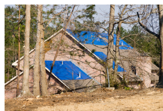
Blue roof covered
