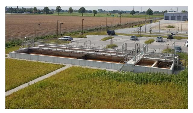
CUSS was nominated as a general contractor for the design and construction of an effluent treatment plant for a producer of dairy products in the south-eastern part of Germany. A main focus was on the civil works of the operational building and the required concrete process tank. The civil works was in full responsibility of CUSS next to the mechanical and electrical installation as well as the commissioning of the plant.
